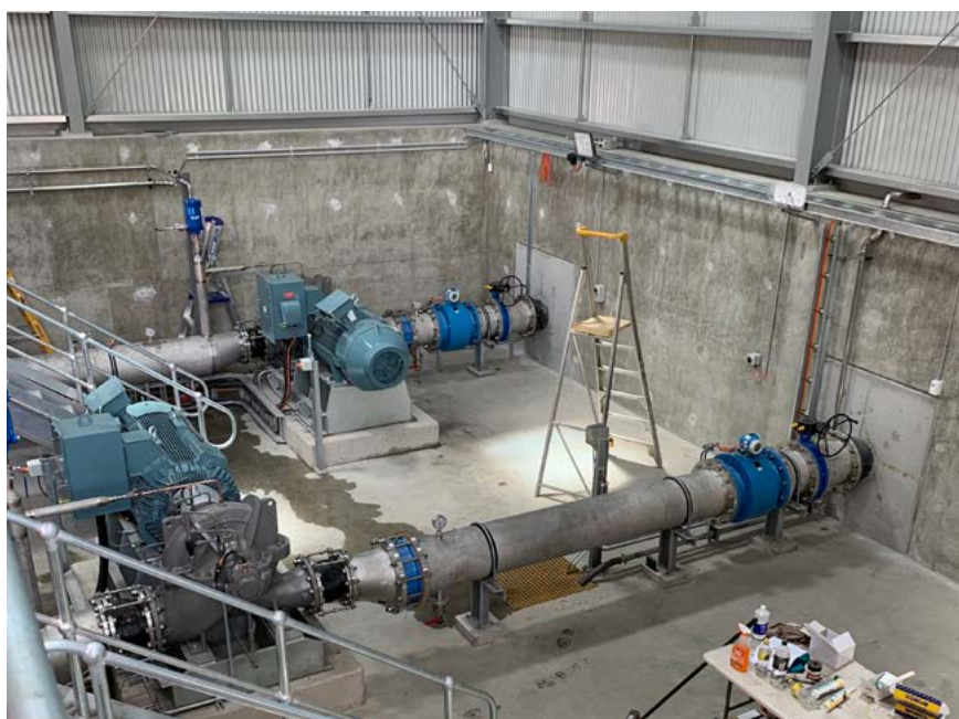
Commissioning of the North East Water Raw Water pump station, installation location of the Promag W 300 0 x DN flowmeter.
