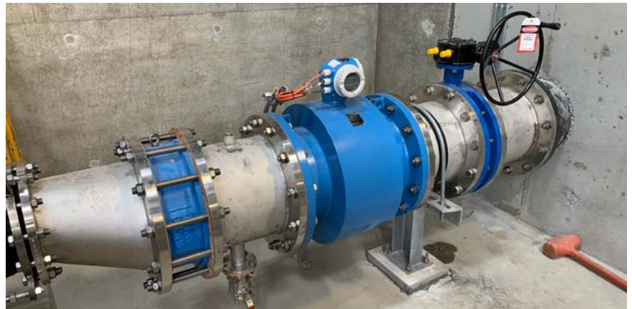
Endress+Hauser Promag W 300 (DN400) 0 x DN full bore flowmeter installed downstream of DN300 to DN400 expansion joint and directly upstream of a DN400 gate valve.
